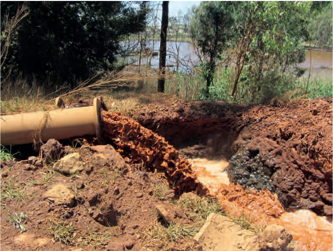
AMD neutralized at the West Rand Treatment Plant has flowed for several years through this pipe and manmade trench to a nearby pit, where heavy metals have precipitated. The water, which has continued on to the Tweelopiespruit in the background, however, has retained dangerously high sulfate levels. © 2014 Bonnie Docherty/IHRC.
